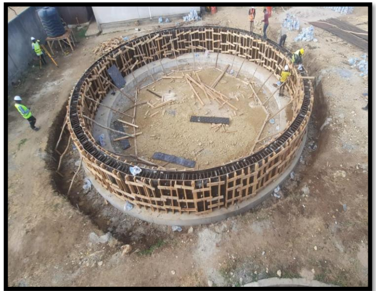
OILCOM TANK FOUNDATION INPROGRESS
