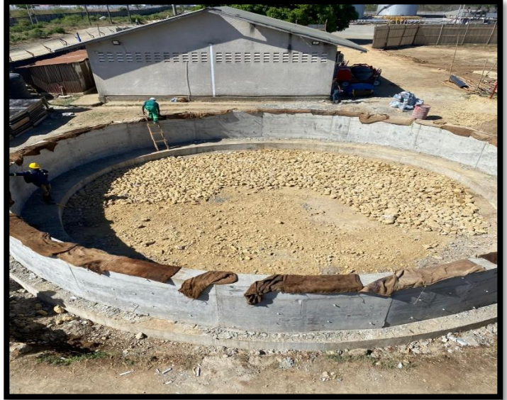
OILCOM TANK FOUNDATION INPROGRESS
