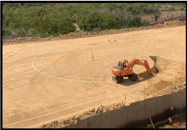
OILCOM TANK FOUNDATION INPROGRESS
