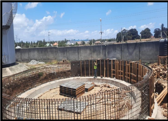
OILCOM TANK FOUNDATION INPROGRESS
