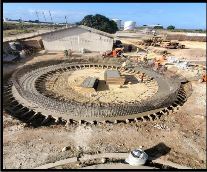
OILCOM TANK FOUNDATION INPROGRESS
