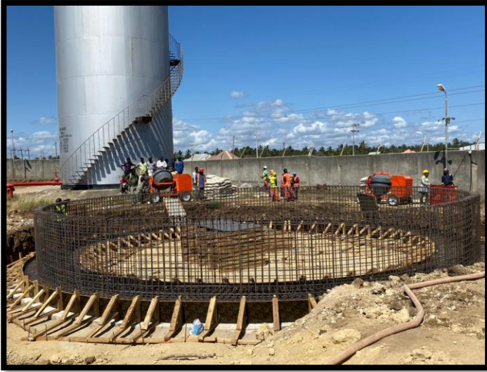
OILCOM TANK FOUNDATION INPROGRESS
