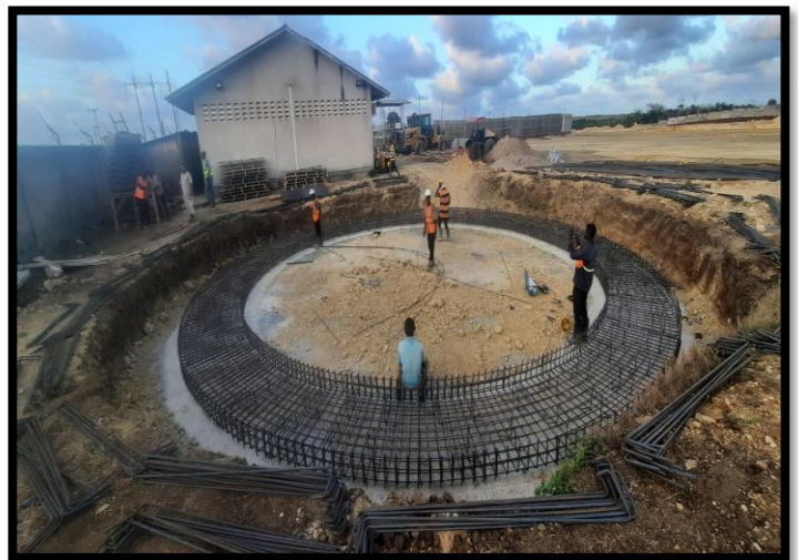
OILCOM TANK FOUNDATION INPROGRESS
