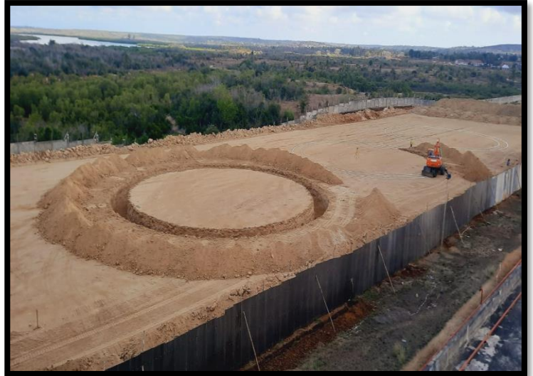
OILCOM TANK FOUNDATION INPROGRESS
